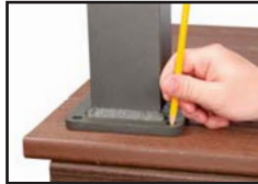
Mark and Pre-drill Holes
