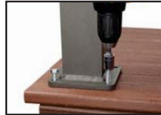
Fasten Post to Deck Surface
