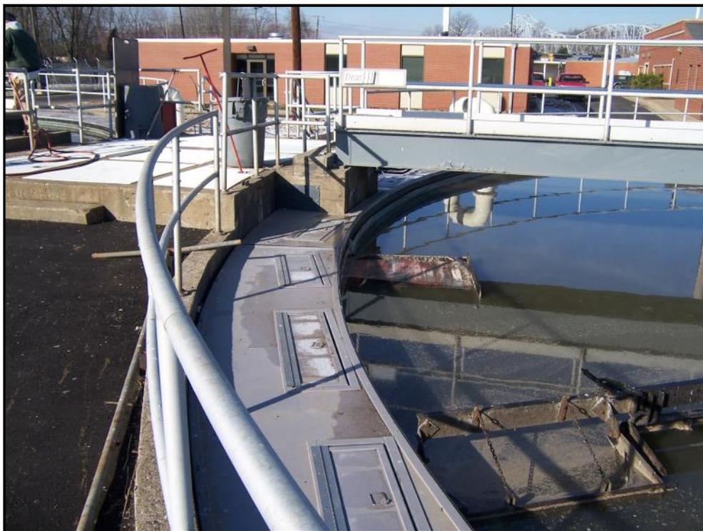
Here shows a Launder Cover opening above an Odor Control Cover. Depicted as a sealed application with Fiberglass plates installed to accommodate wall opening also provides hanger supports for cover.
