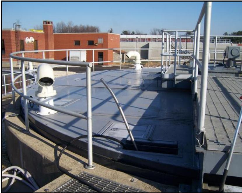
Full Odor Control Cover over Thickeners at Parkesburg, WV WWTP with Integral Access Hatches to all of the primary maintenance areas.
