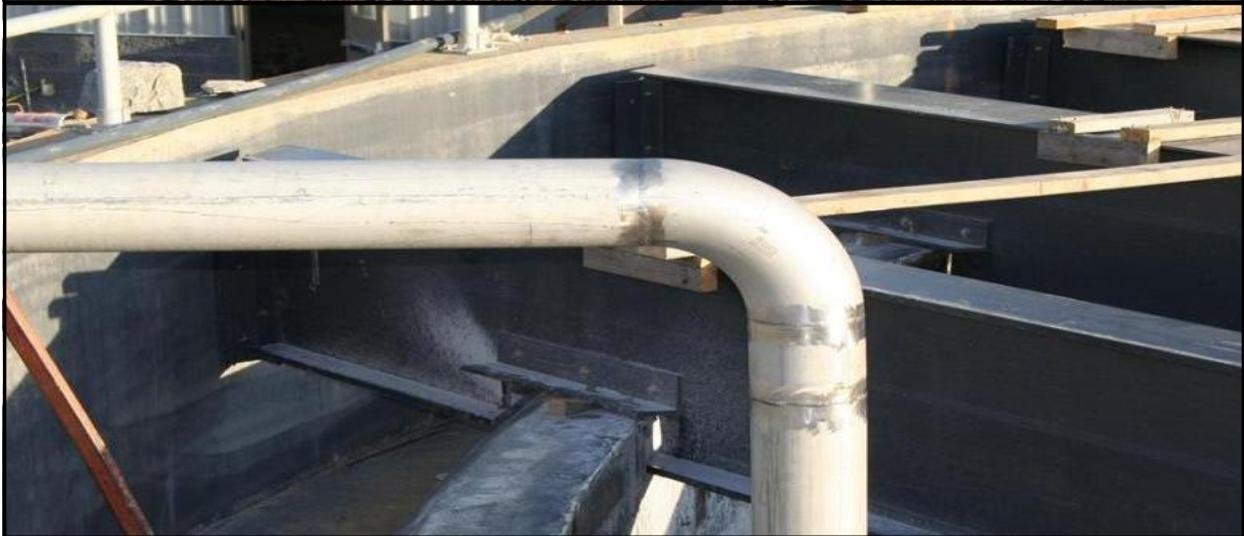
Fiberglass Structural Support framing for full tank odor control cover at Wolf Creek WWTP Abington, VA.
