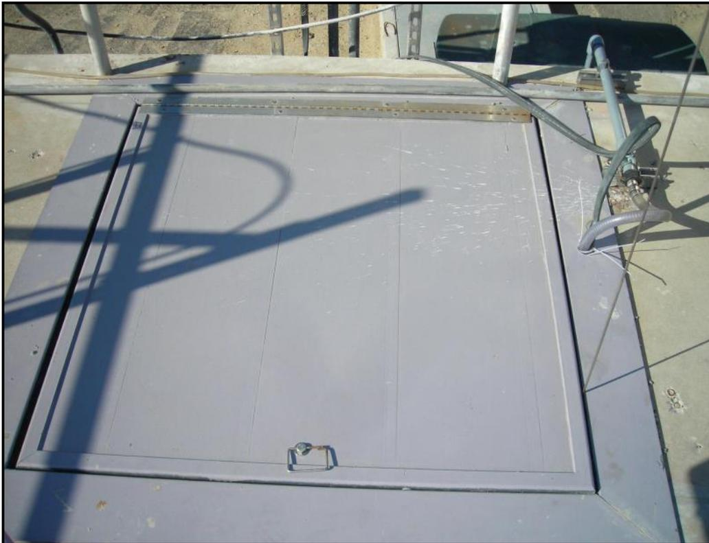
This flat drop in floor access door is also installed in Ontario, CA. The flange around the opening is 6" x 6" x 1/4", and can be recessed if a form out is done prior to installation or it can be set in as is without creating a tripping hazard. This door was installed in an existing structure. This door also can be provided sealed or not sealed.
