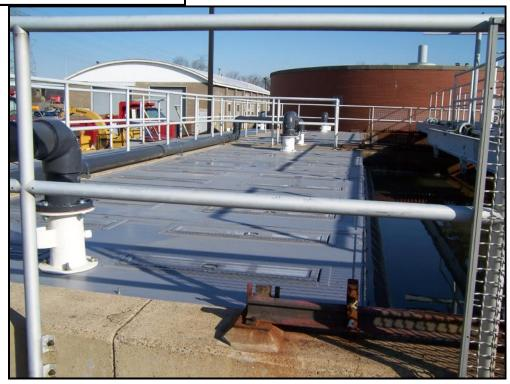
Shown is Flat Covers over Effluent Trough with Integral Doors to access weirs for maintenance. At one end of this Control Cover the wall angle edge. The opposite end of the cover is supported by fiberglass plate columns and also can work as a seal surface.
