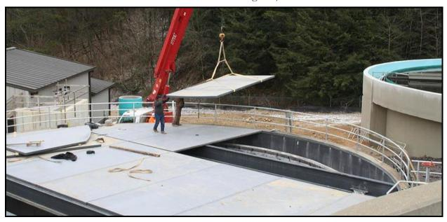
Fiberglass Cover panels being installed for above
