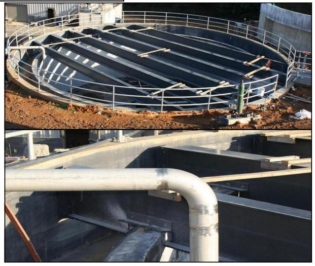
Fiberglass Structural Support framing for full tank odor control cover at Wolf Creek WWTP Abington, VA.
