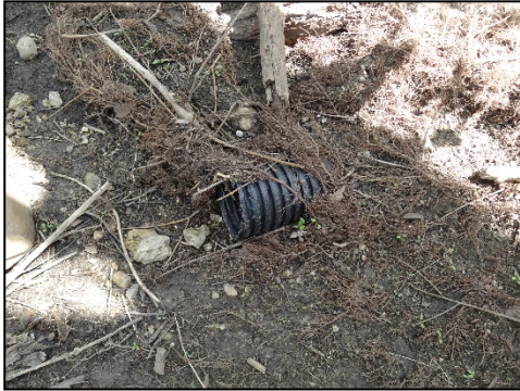
Drain tile outlet into Somers Branch from the south field at Gitzlaff,
