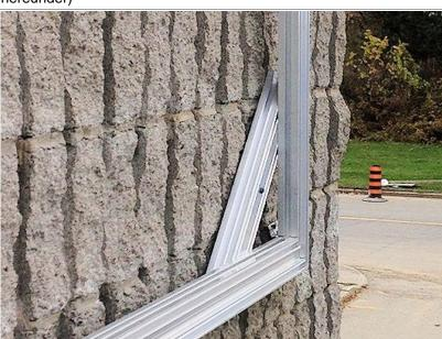
In the corners a piece of TS44 was inserted to both fix the frame on this rough wall and reinforce the corner rigidity.
