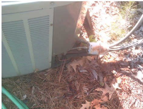
Heat pump sitting directly on the ground.
