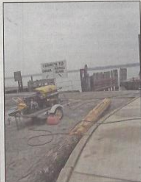
The replacement for the broken pylon
