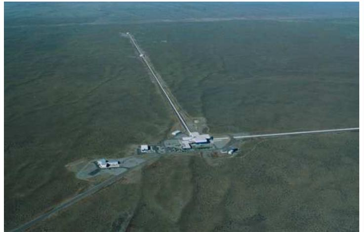
*Figure 1. The right angle oriented laser tunnels of the Hanford LIGO interferometer.*
