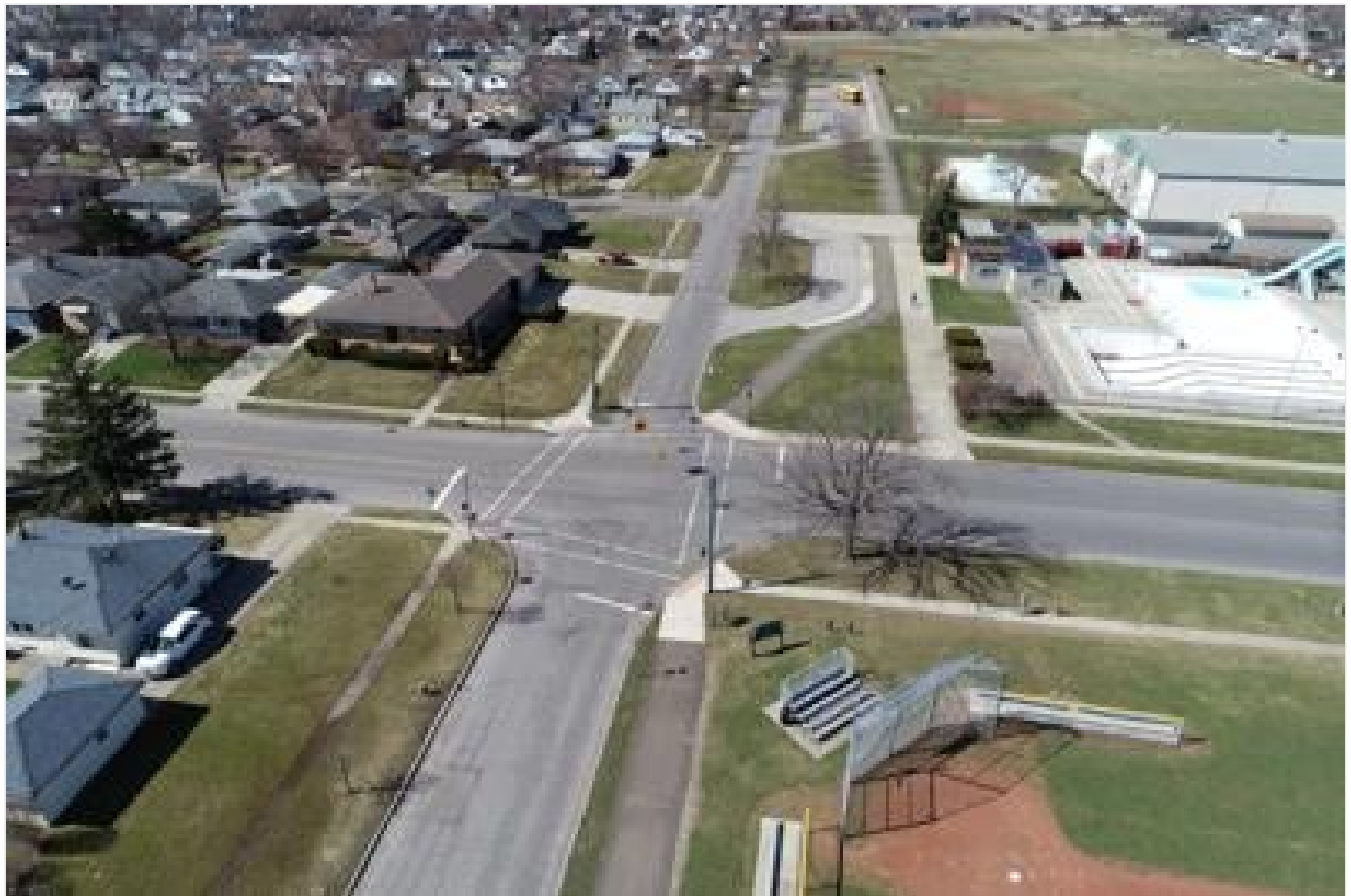
Work begins on $1.3M Town of Tonawanda roundabouts
