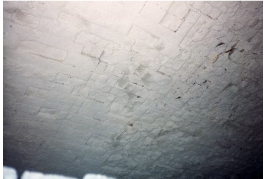
Ultra-Z sprayed over IFB
