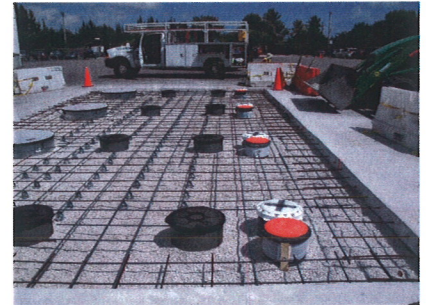
Underground Tank Upgrade at Budget Car Rental
