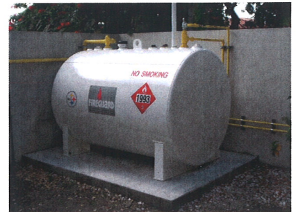
Above Ground Fire-Rated Generator Fuel Tank
