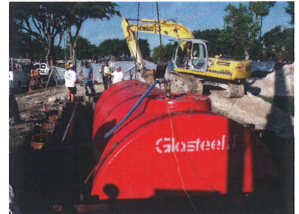
Installation of New 15,000 gal Underground Double-Wall Fuel Storage Tank for Generator System
