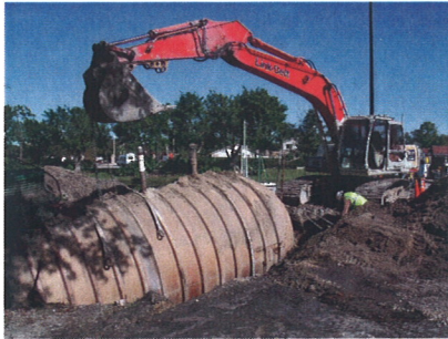
Removal of 15,000 gal Underground Fuel Tank at West Boca Medical Center
