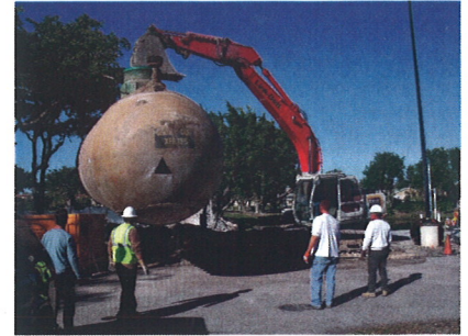
Removal of 15,000 gal Underground Fuel Tank at West Boca Medical Center
