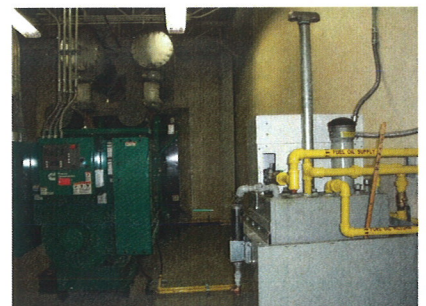
Above Ground Fire-Rated Generator Fuel Tank
