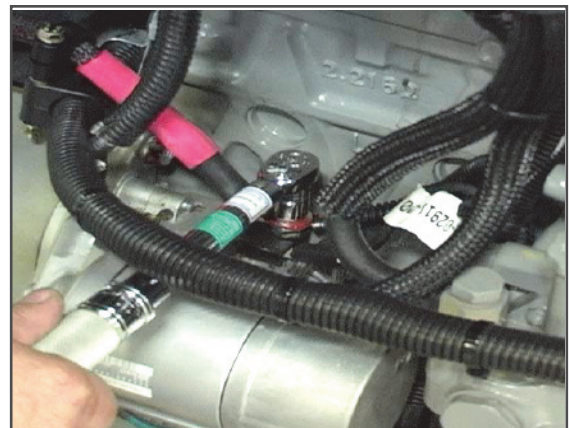
Figure 8.60 Positive Starter Wire Installation
