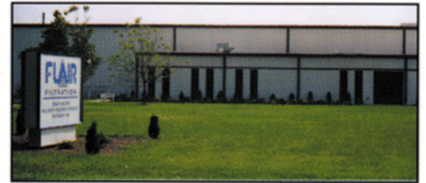
Flair Filtration Plant at Stanley, North Carolina
