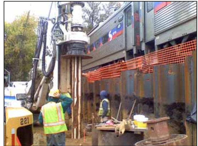
Ryers Station Reconstruction
