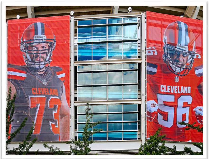
Cleveland Browns Stadium Two of eight 22'x 42' TS32 frames with mesh banners
