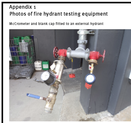
Figure 10 – External Hydrant Test Arrangement
