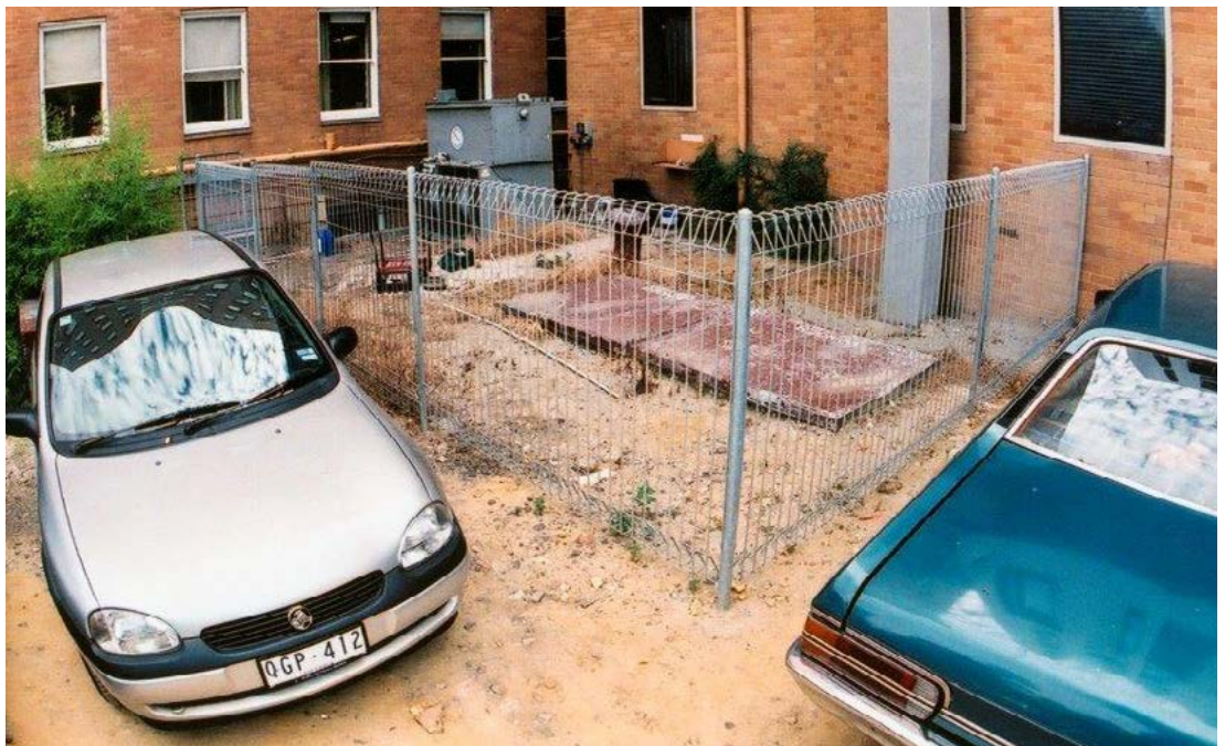
Environmental contamination: An unmade car park in the area adjacent to a cooling tower may increase the levels of solids in the water and must be addressed in the RMP
