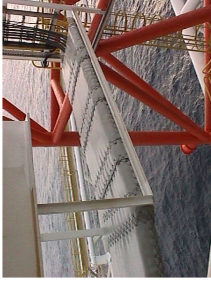
Flexible PFP jacket on cable tray
