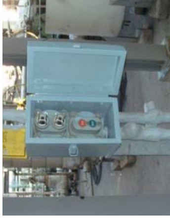
Epoxy PFP box for electrical controls
