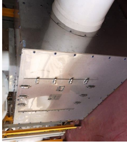
SS enclosure for offshore safety valve
