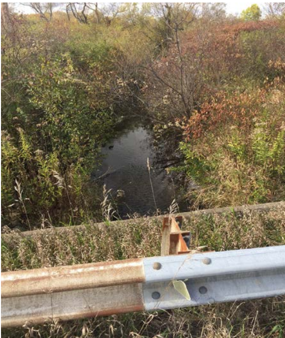
Figure 50. Elk Creek at Sparks Road bridge looking upstream.
