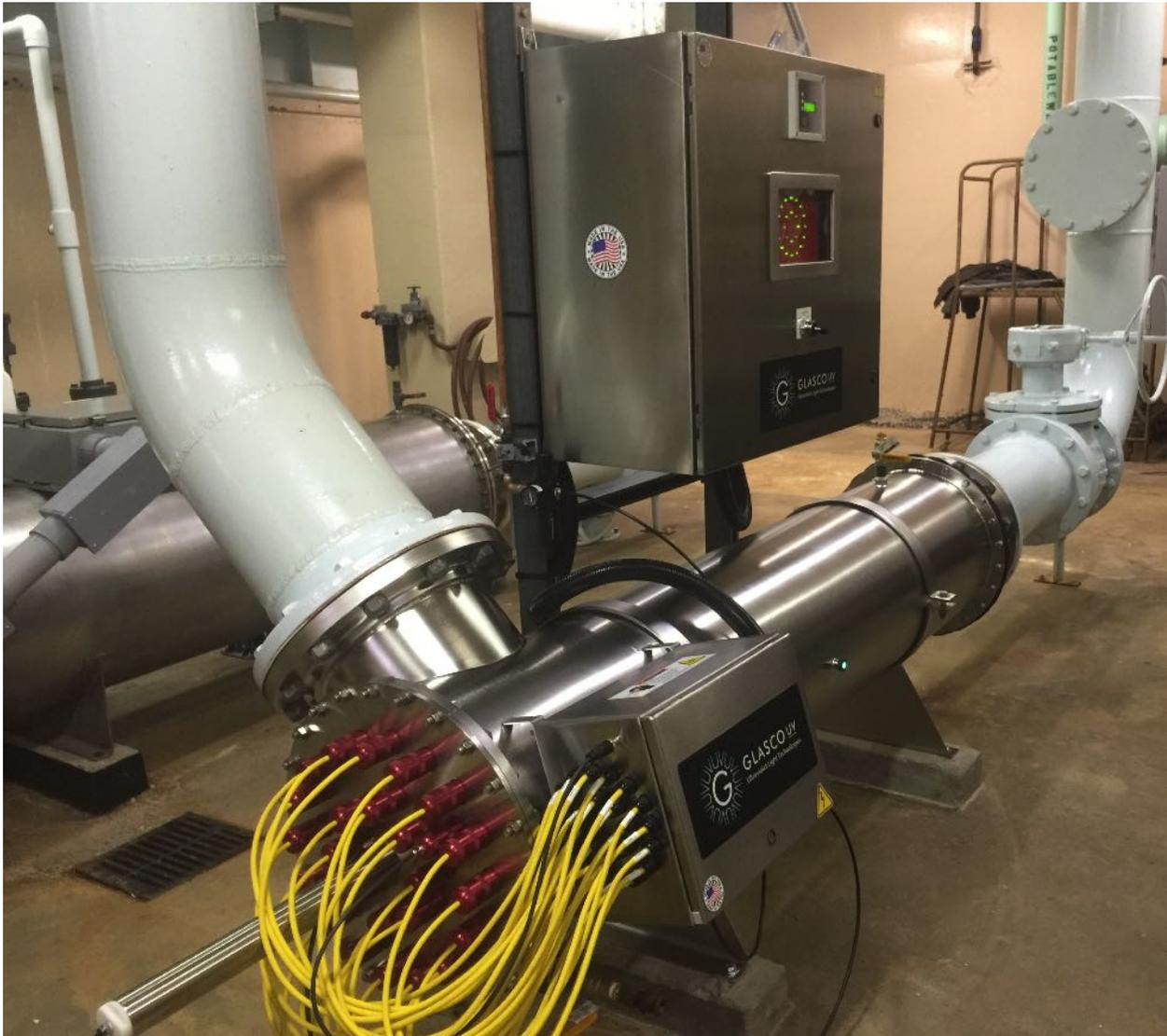
Chambered UV disinfection systems have been used to treat secondary wastewater since the 1980s. The US EPA indicates that over 50% of the first UV wastewater systems were chambered.
