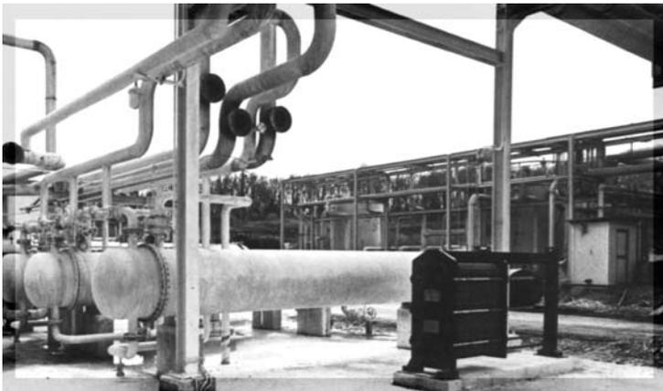
Figure 30. Picture of Series R405 Paraflow being installed.
