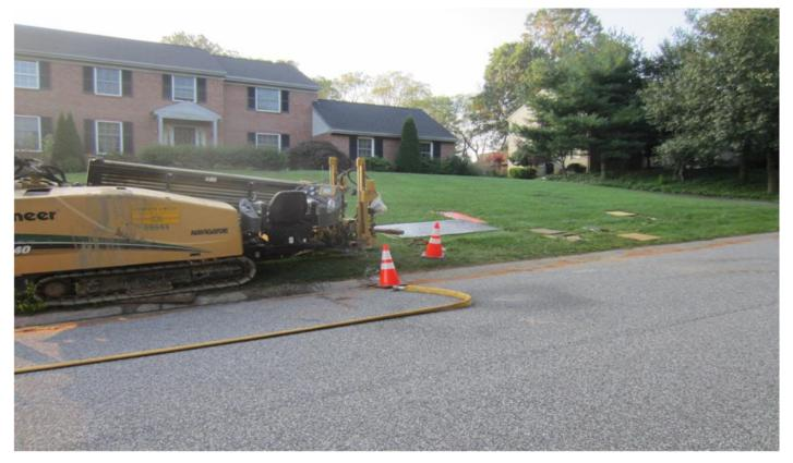
Install new main throughout neighborhood in the state right-ofway at the curb line utilizing a directional bore technique.
