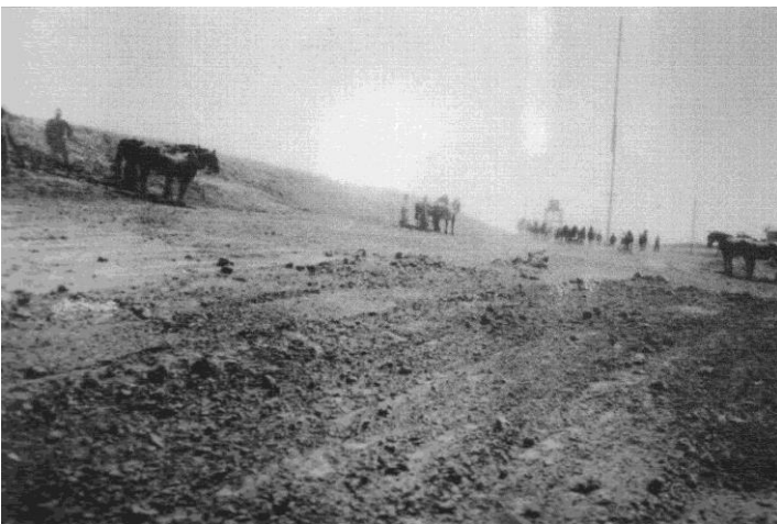
Grading a levee with Fresno Scraper
