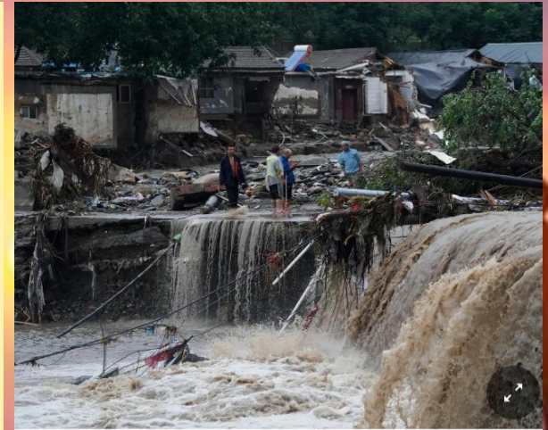
Floodwater damage on the outskirts of Beijing. Andy Wong/Associated Press
