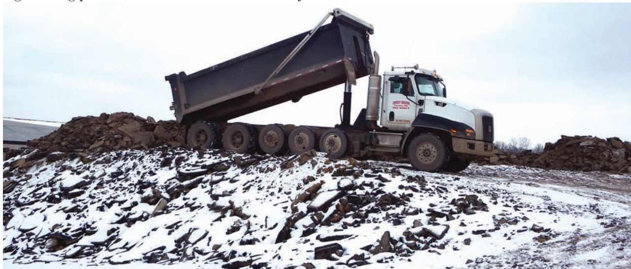
One of the 100 plus loads of asphalt tear out that was expected to be brought in on the day of our visit, arrives at the top of this stockpile of material and is dumped in a safe location.
