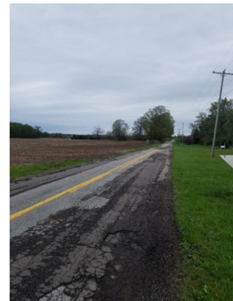
Pictures showing the poor condition of 71 st St. because of an inadequate prior drainage system
