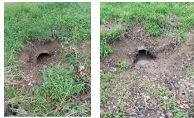
Examples of the private, non-connected drainage system that existed prior
