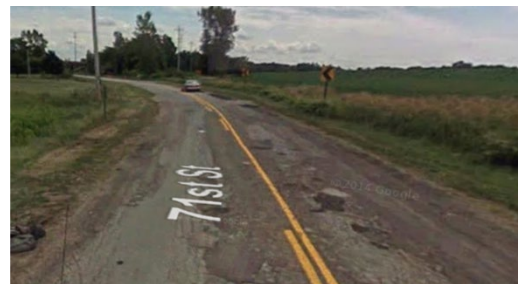
Pictures showing the poor condition of 71 st St. because of an inadequate prior drainage system
