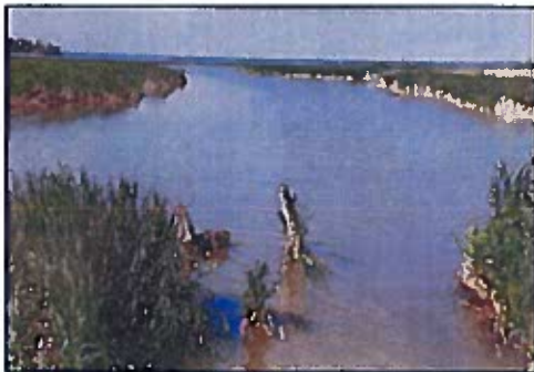
Photo 2: Remains of the old weir, June 2018.
