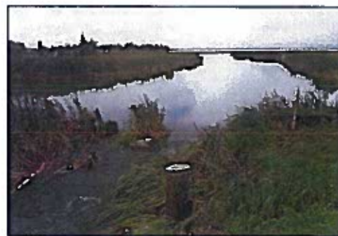
Photo 3: Remains of the old weir, August 2018.
