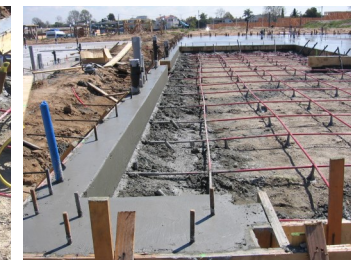
5. Permanently leave the lower portion of VaporStake™
