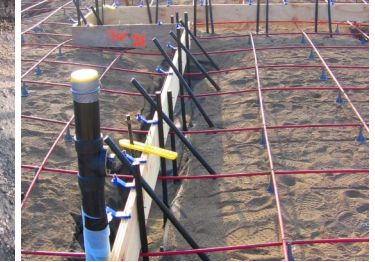
3. Using duplex nails, nail forms directly to VaporStake™
