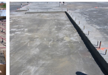
6. Finish slab over VaporStake™
