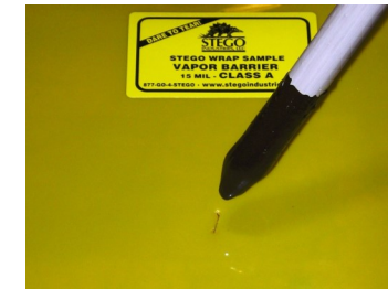
1. Dip the pointed end of the VaporStake™ into the mastic that is provided by the vapor retarder.
