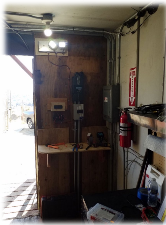
☀ 10/25/2019 The 4C's repeaters & original battery connected to the new solarized battery and separated from PG&E source
