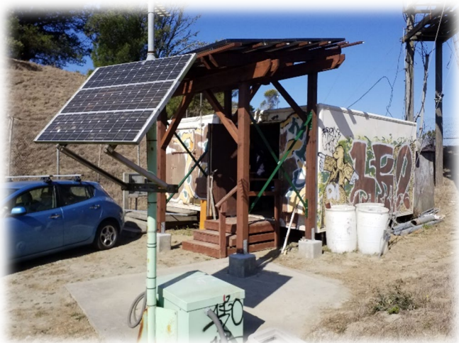
▼ 10/13/2019 Solar modules mounted and ready to connect to new battery
