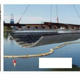
In the top left image, mattress sections are filled with stone (stone size varies) and the geogrid is seamed shut. In the top right image, REACTIVE CORE MAT® is attached to the bottom of the mattress. The REACTIVE CORE MAT® is filled with Organoclay®, which is used to adsorb contaminants. The mattress system's subaqueous installation is aided by divers to ensure proper positioning of the mattress sections.
