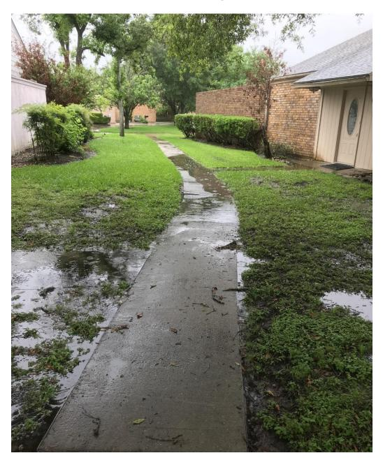
10 – Drainage/Concrete, 63 & 62 Chervil Common Sidewalk Replacement. It Stays Covered in Water When Ground Is Saturated. Estimate \$630
