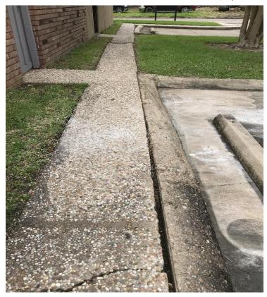
49 – Street, Caulk Joints At Various Sections Of Streets In Order To Prevent Rainwater From Washing Out Supporting Soil Which Allows Concrete To Break; Estimate \$6,000
