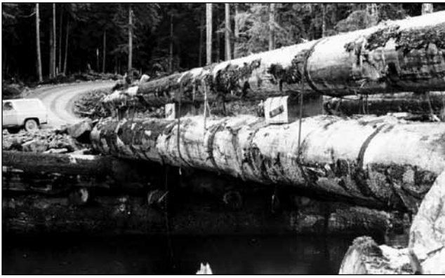
Figure 6–5. Logs are used to construct logging bridges in remote forest areas.
