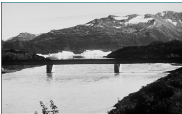
Figure 17–9. Glulam beam bridge over the Dangerous River, near Yukatat, Alaska, consists of three 43.5-m (143-ft) spans. Each span is supported by four 2.3-m (91.5-in.-) deep glulam beams.
