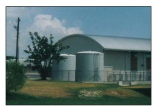
Water collected from the roof of the J.J. Pickle Elementary School and St. John Community Center is stored in three large tanks behind the building and used as cooling water for the complex's airconditioning system.
