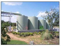
The H-E-B at the corner of Brodie Lane and William Cannon Blvd. in south central Austin irrigates an adjacent landscape of water-thrifty plants with rainwater stored in four painted steel tanks totaling 28,000 gallons. A 24-inchdiameter pipe conveys water from the roof to the tanks.
