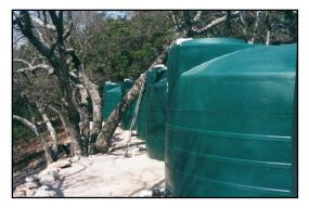
Figure 2-6. Low-profile 5,000-gallon polypropylene tanks
