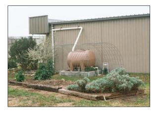
Rainwater captured from the 1,500-square-foot roof of the Walker County Extension office is stored in a 550-gallon polypropylene tank, a type readily available at ranch supply retailers. The 10-gallon flush diverter is the vertical standpipe visible to the left of the tank. Captured rainwater irrigates an adjacent Master Gardener demonstration garden, foreground.
