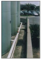
Tanks are linked with 6inch PVC pipe. Valves allow taking one or more tank off-line for draining or cleaning.
