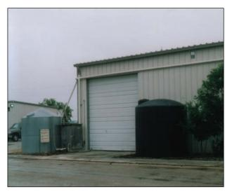
As a demonstration project, a 750-gallon galvanized steel tank captures rainwater from the 5,000-square-foot roof of the Hays County Extension Office.
