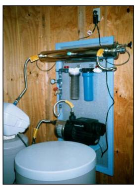
Figure 2-12. Typical treatment installation of an on-demand pump, 5-micron fiber filter, 3micron activated charcoal filter, and an ultraviolet lamp (top).
