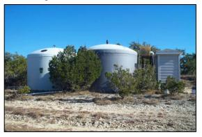
Figure 2-5. Two 10,000-gallon fiberglass tanks
