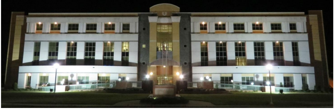
Sutton Administration Building (Credit: John Zheng)
