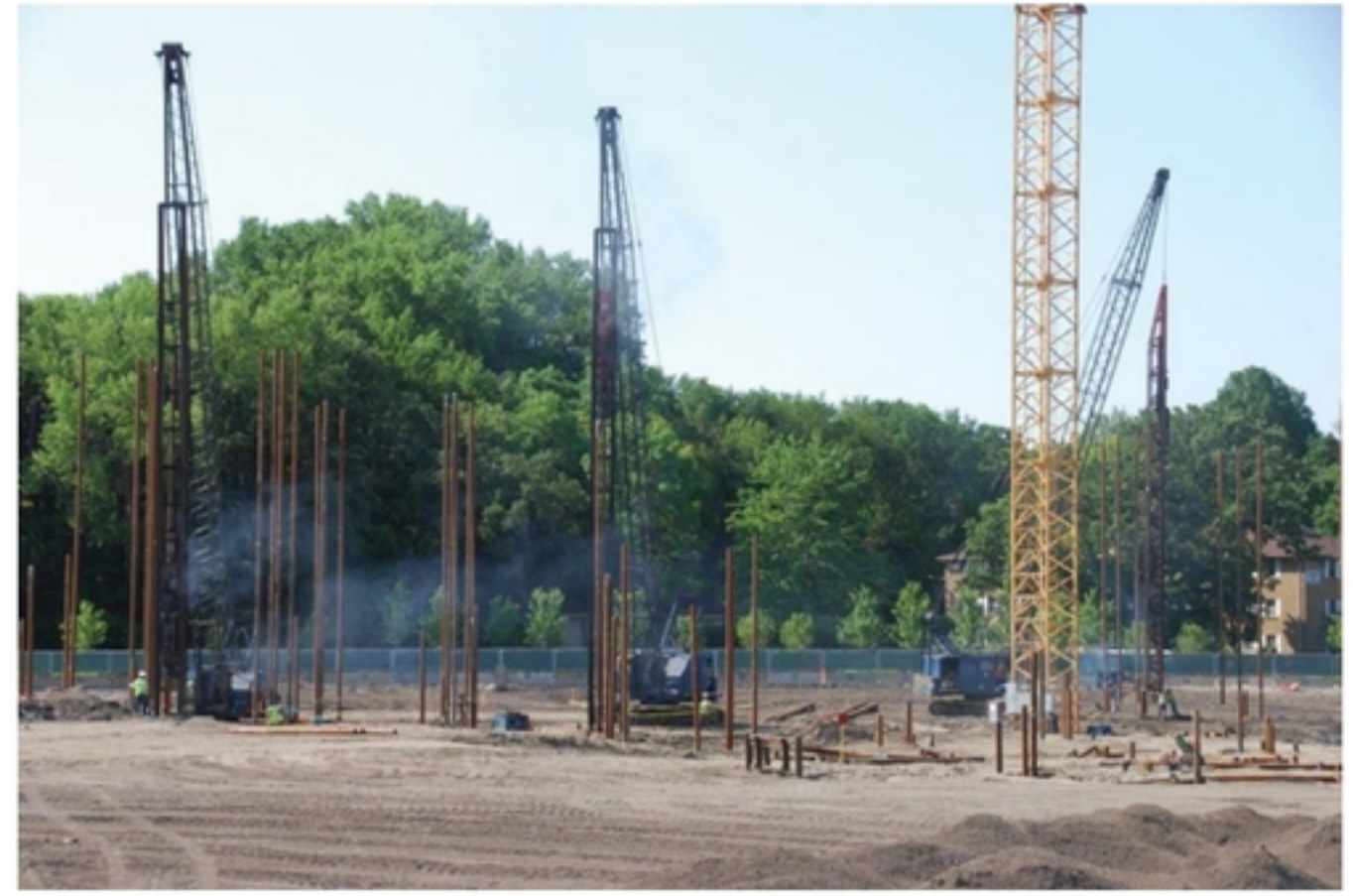
Production pile installation
