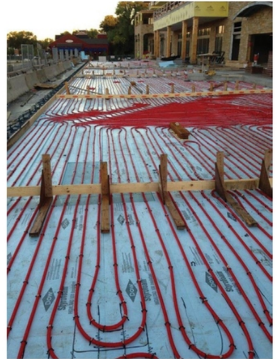
Snow-melt tubing was placed in sidewalk and driveway areas
