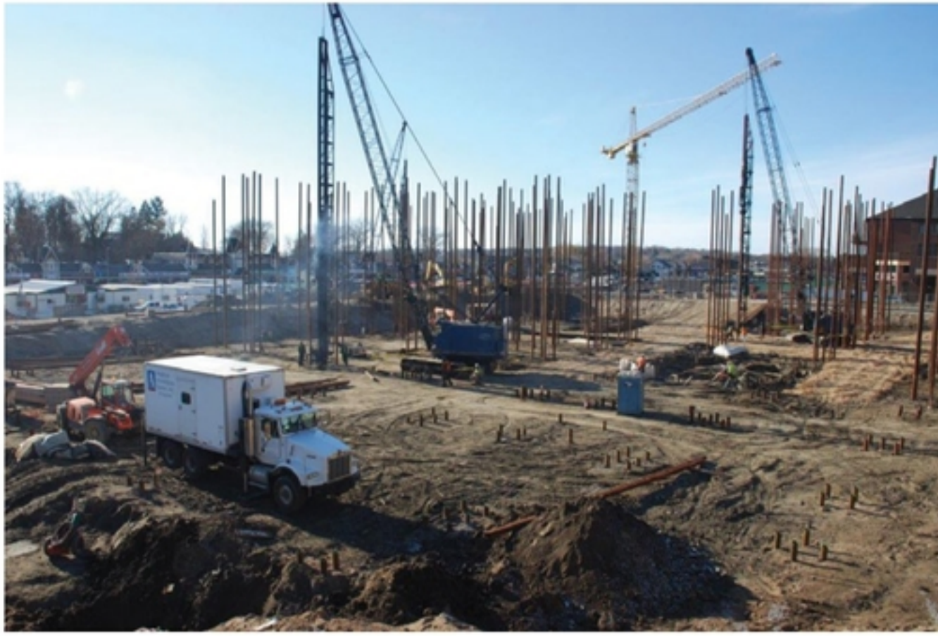
CPT soundings confirmed conditions in uninvestigated areas during construction
