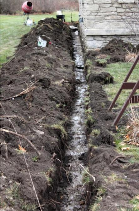
The drainage project was a big job. Exposed bedrock slopes toward the street. The system is now locked into the village storm drain, which should handle the ground water issue.
