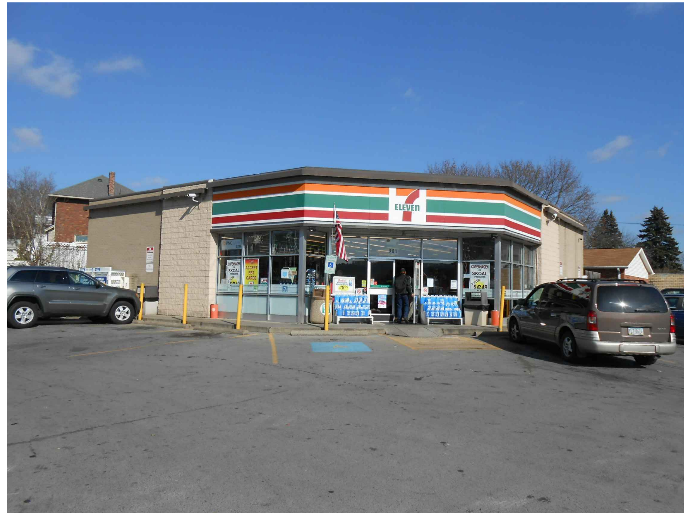
EXISTING SITE PHOTOGRAPH
