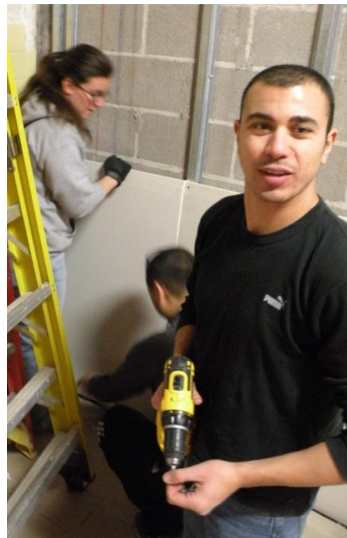
Above, members of Echo Team install sheetrock and plywood.
