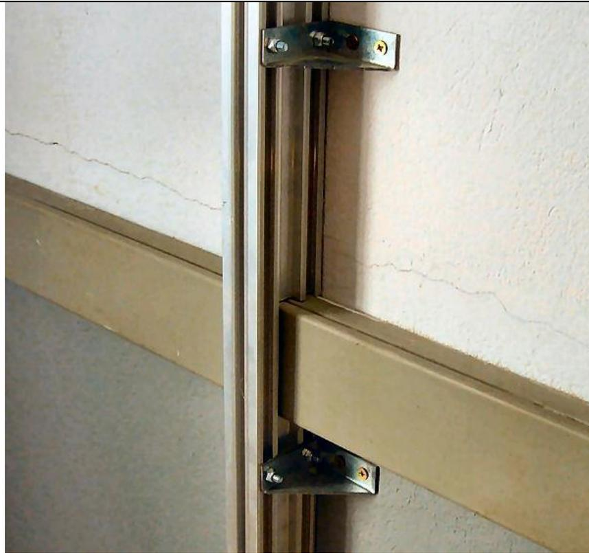
Example of fixation of a frame using 2" reinforced brackets.
