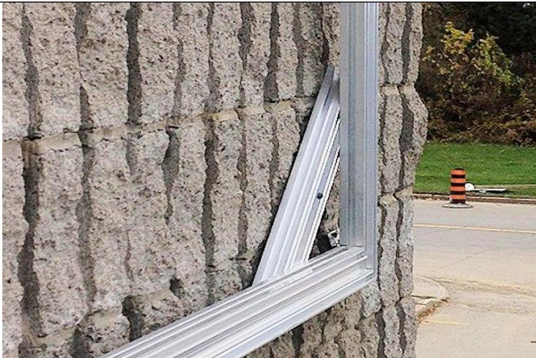
Example of a frame corner screwed on top of a piece of TS44 extrusion to avoid contact with the rough stone wall. This installation could be used for the four corners of your project.
