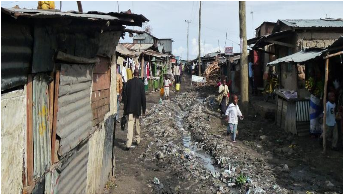
Plate 4 : Obunga Informal settlement in Railways ward
