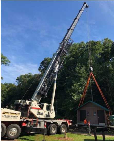
The restroom is being set in place...
