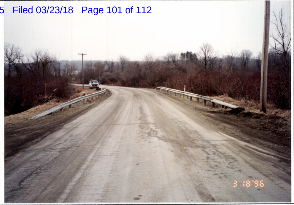
LOOKING SEGMENTS BACK
