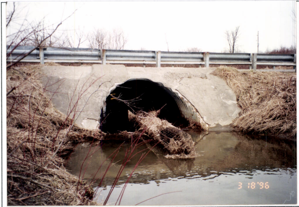
LOOKING @ RIGHT SIDE INLET
