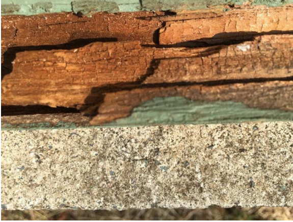
Figures 3 and 4. Wood failure due to termites (left) and rot
