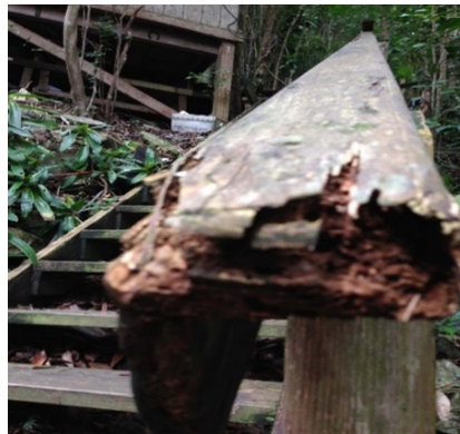
Figure 2. Railing added in 2011 to stairway built in the 1980's
