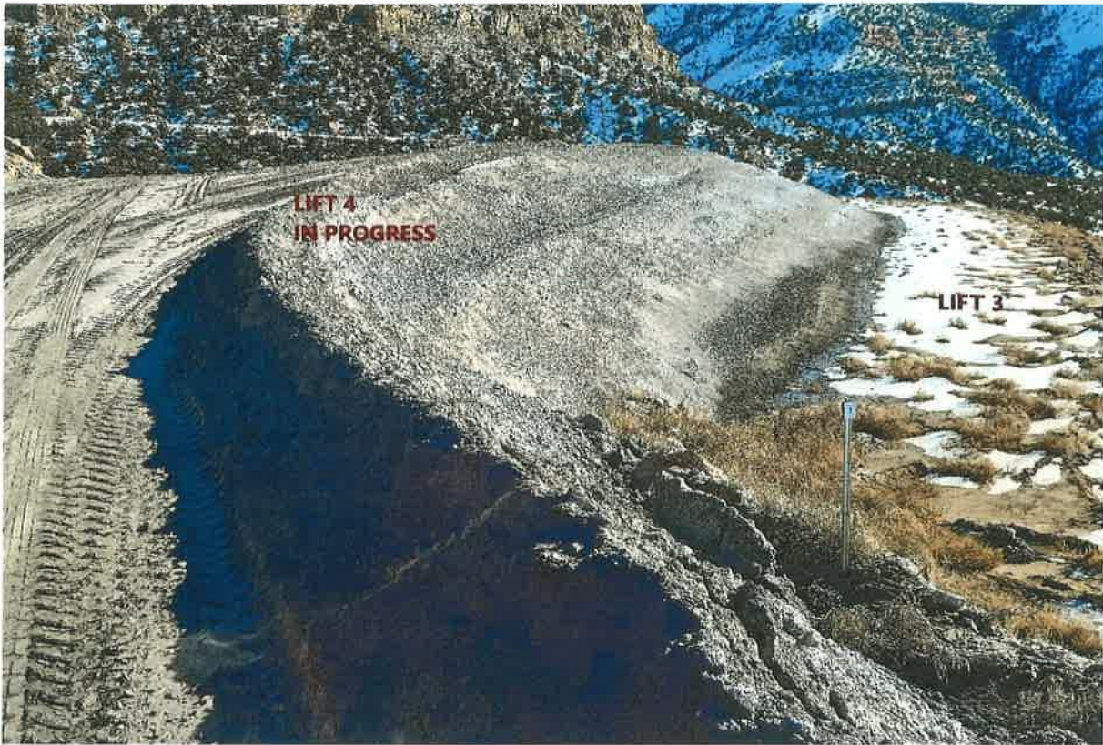
Surface of Lift #4 in process – photo looking south-southeast
