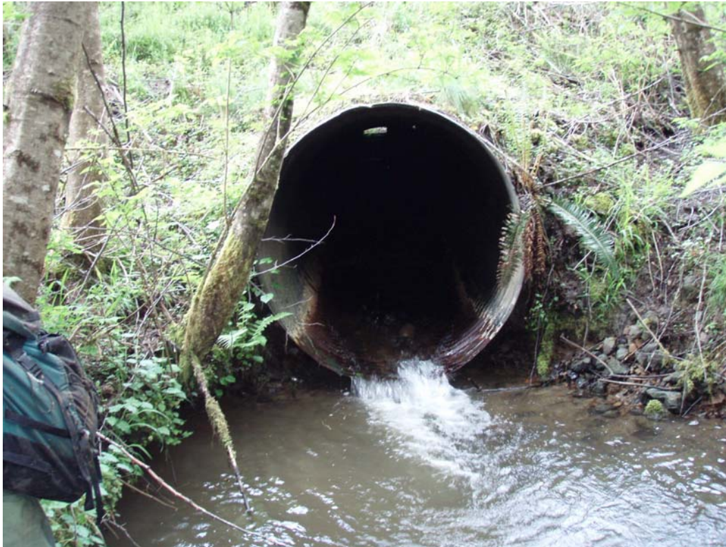
Figure 3.45. Photograph looking upstream at partial barrier culvert in unnamed tributary 19.0135.
