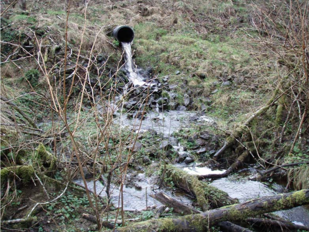
Figure 3.46. Photograph looking upstream at culvert out fall on unnamed tributary WP 203.
