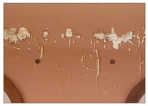
Interior damage done by water leaking in from cracks caused by damaged limestone exterior.
