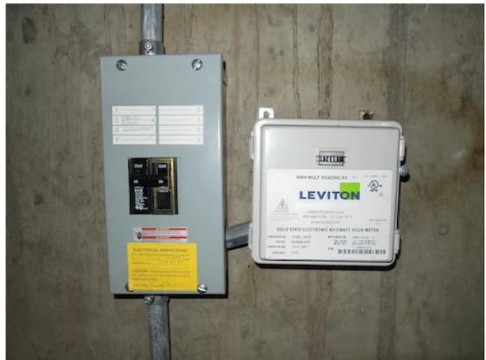
**PEV Charging plans and infrastructure:** One Leviton Level 2 EVSE (50-amp circuit).
