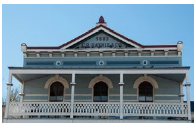
10. Balcony Structure Barbara Hunley
