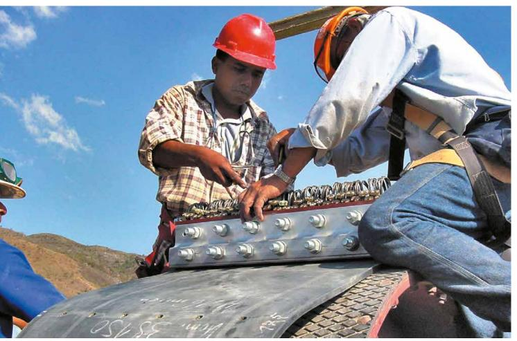
Splicing of steel-reinforced belt
