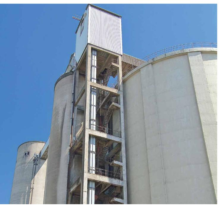
Bucket Elevator for cement silo feeding
