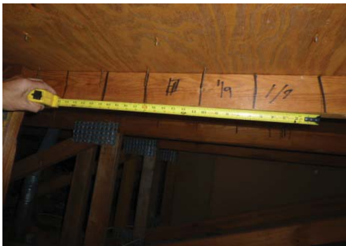
#3 ROOF DECK ATTACHMENT
