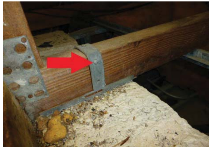
#4 ROOF TO WALL ATTACHMENT OPPOSITE SIDE
