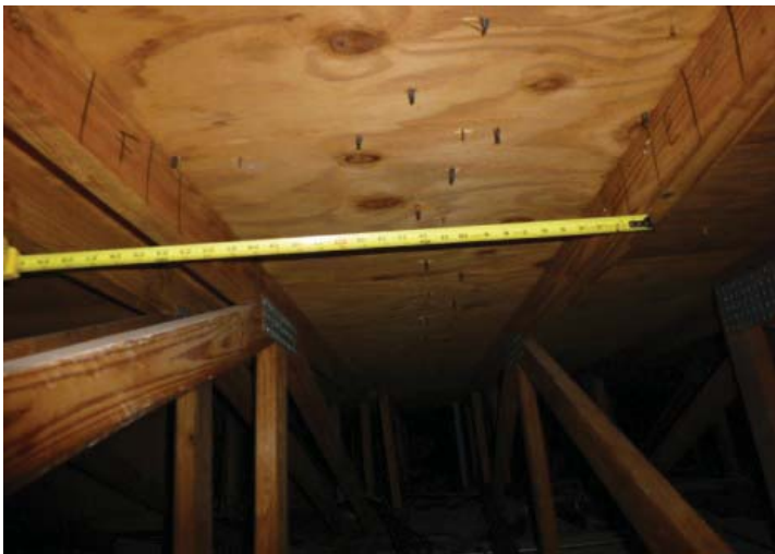
TRUSS/RAFTER SPACING
