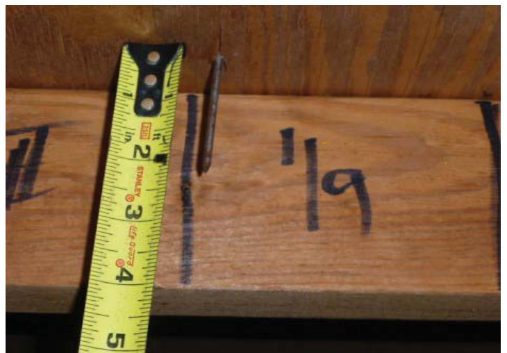
#3 ROOF DECK ATTACHMENT
