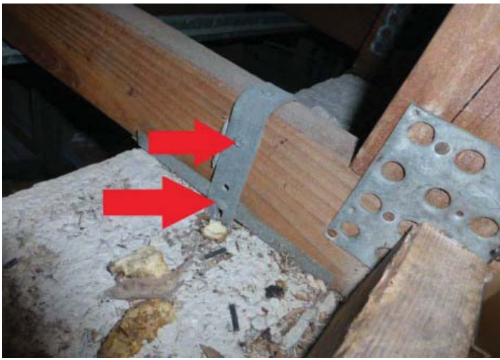
#4 ROOF TO WALL ATTACHMENT FACE SIDE
